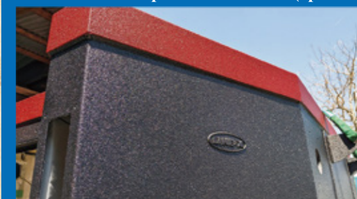
First in Japan !! High-purity polyurea coating applied to nuclear shelters in April 2023. Other high-purity polyurea coatings also utilized.
